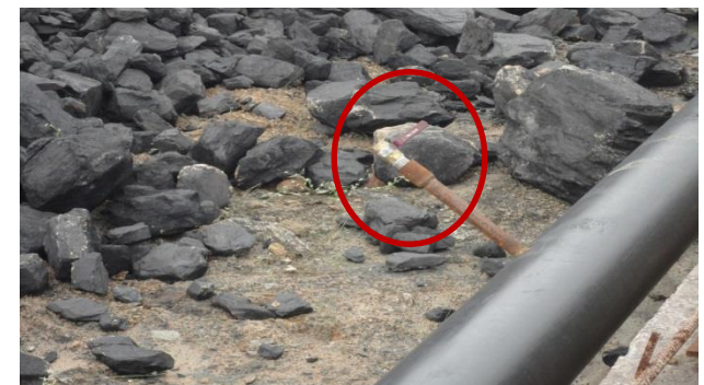
Fixed type DS system at Coal Yard
