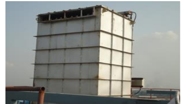
Fixed type DS system at Coal Yard
